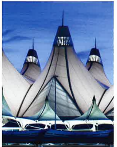
FIGURE 2.5.8c: Denver International Airport is made from fibreglass.
